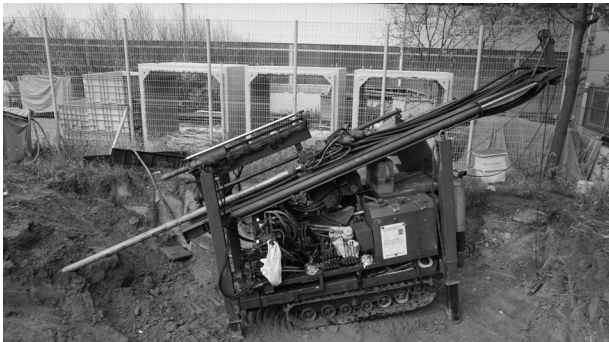
Fig. 4. Angular drilling with a hydraulic rotary drill (D & B-10D)
