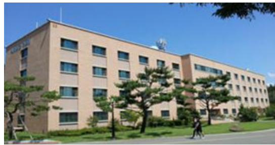
Fig. 1 View of a experiment building
