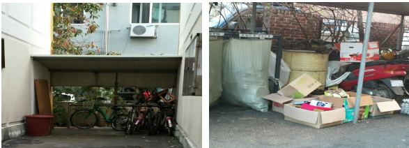
Fig. 6. Lack of parking area in old aged apartment
