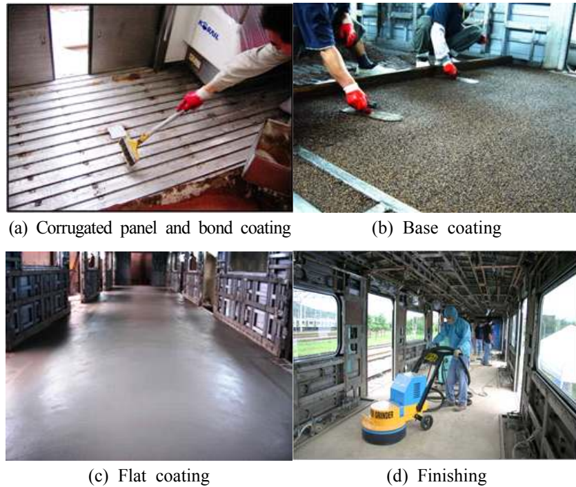
Fig. 2 Process of Unitex construction
