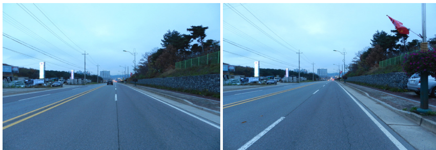
Fig. 2 Road accident site
