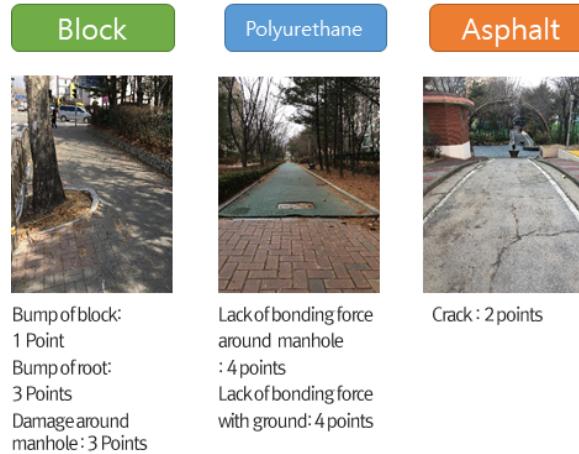
<Fig. 4> Pavement surface evenness survey results
