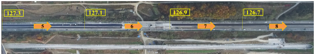
〈Fig. 7〉 Image of work zone by drone(Yeongdong Expressway)
