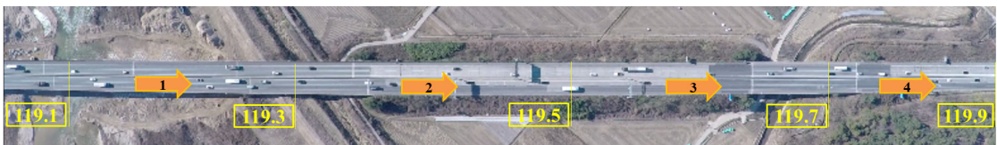
〈Fig. 10〉 Image of WIM system by drone(Jungbu Naeryuk Expressway)
