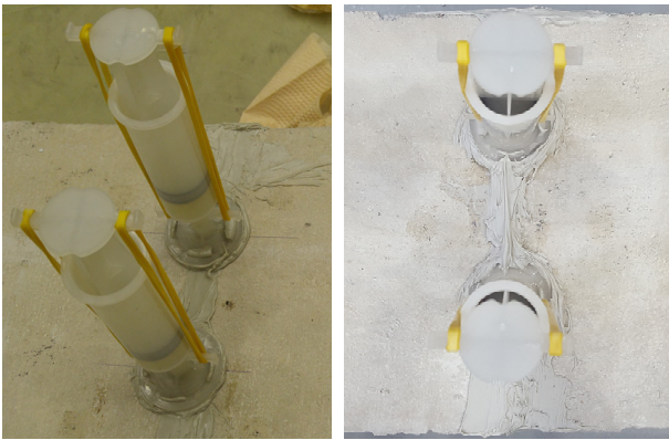
Fig. 4. Crack repairing process using epoxy
