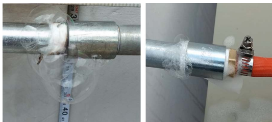
Fig. 5. Leak check with soap bubble.
