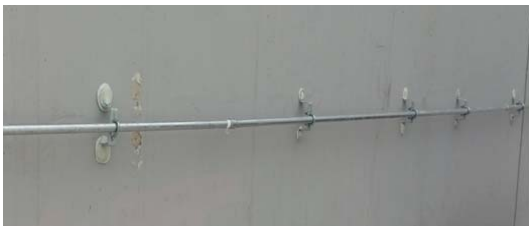
Fig. 1. Pipe installation on outer wall.
