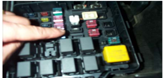
Fig. 3. Installing location for Air conditioner diode.
