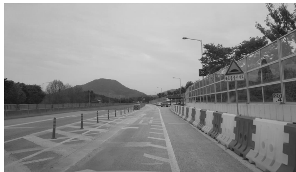
Fig. 3. A Short Entry Connection Roads of the Rest Area for Drowsy Drivers
