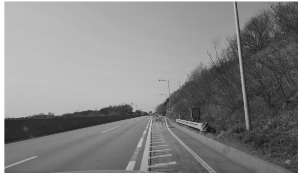
Fig. 2. Decelerating Lane in Which the Entry Part is not Sufficiently Secured
