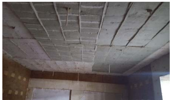
(B) Inside of the Experimental Furnace
