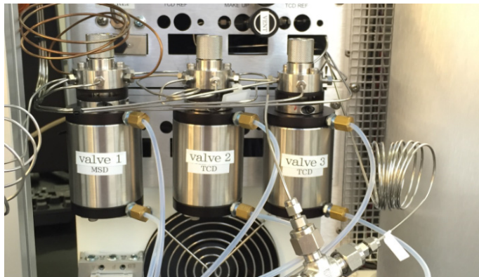
Fig. 3. Three valves installed at the back of GC-MSD/TCD.
