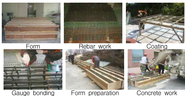
Figure 6. Making process of RC beam using PCS-coated rebar
