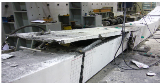
Fig. 17. Failure pattern of BF1.0-32 in central segment
