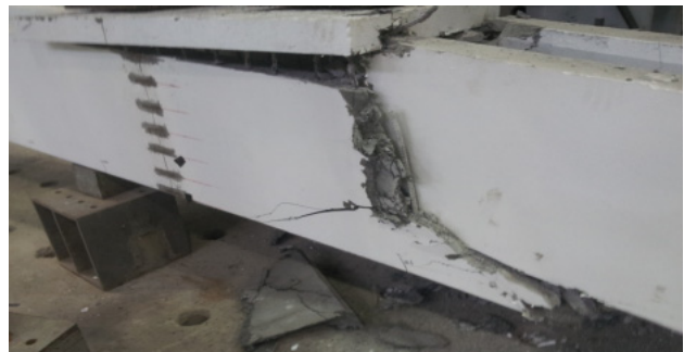
Fig. 16. Failure pattern of UFS0.7
