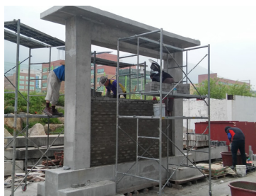
Fig. 2 Masonry wall infill
