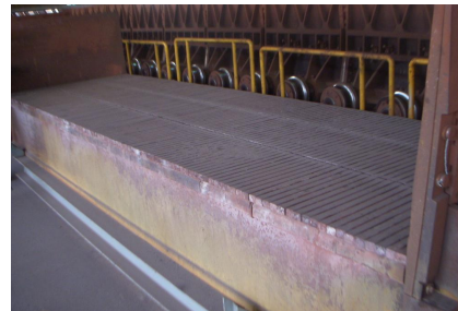
Fig. 2 Grate bar bogie in sintering process
