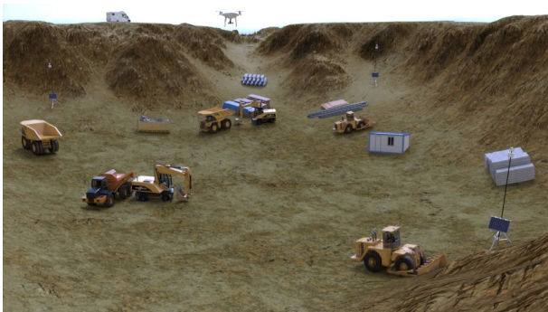
Fig. 2. Fleet Management System for Earthworks (Smart Construction Tech Research Group, 2018)
