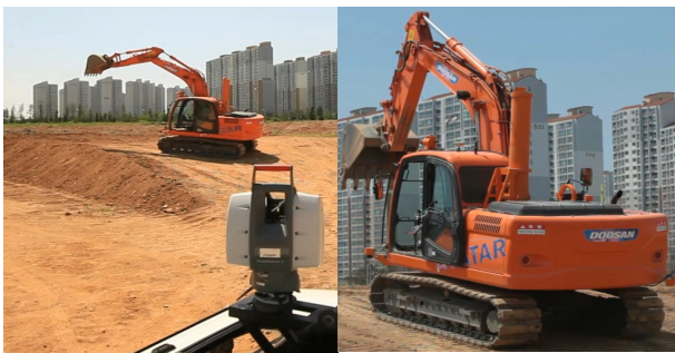
Fig. 1. Unmanned Intelligent Excavator
