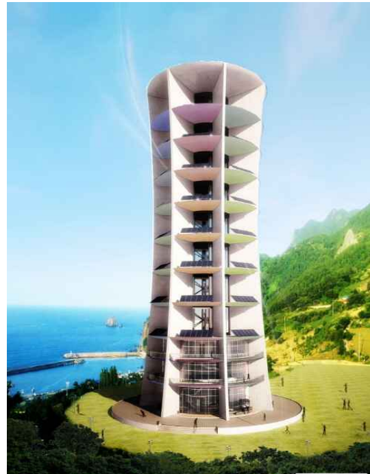
Fig. 1. View of wind power tower with VAWTs
