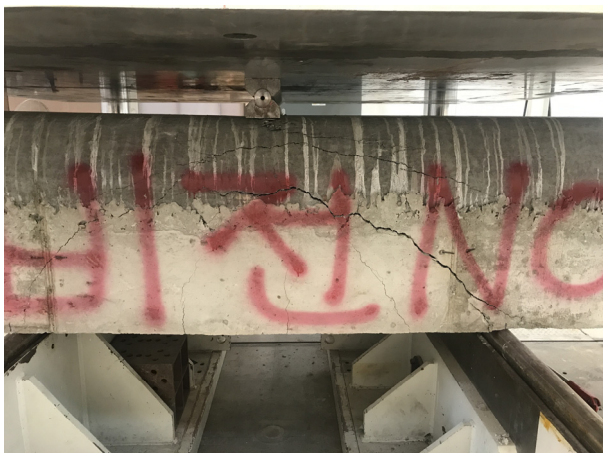
Photo 4. Failures of non-composite additional wall during shear test (N-S-1)
