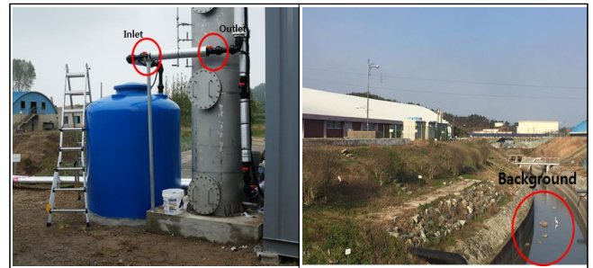
Fig. 1. The sampling point (A turbidity reduction system is installed in the hot water utilization system. The sampling point is shown by a circular solid line).
