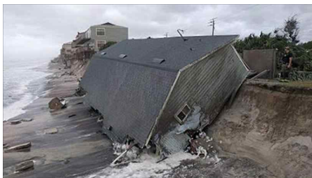
Fig. 4 Lee county damage case2
