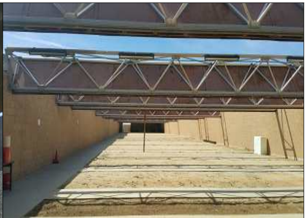
Fig. 2. shooting range facility
