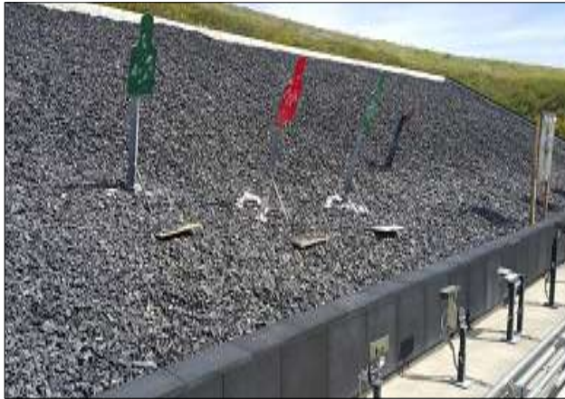
Fig. 7. shooting range facility
