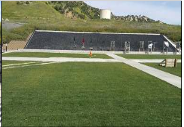
Fig. 8. shooting range facility
