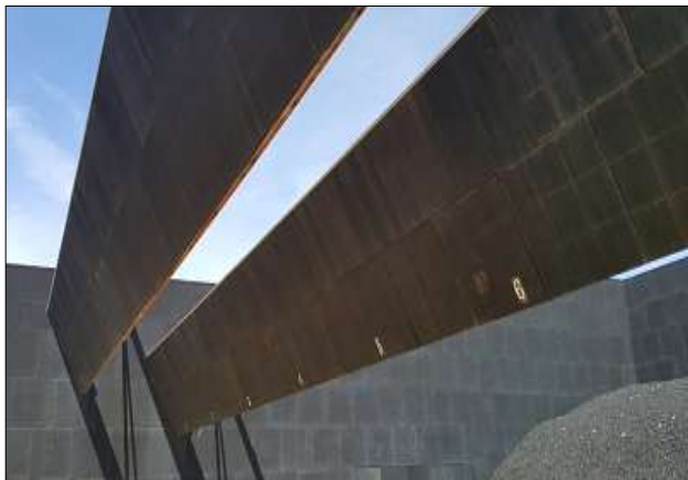
Fig. 1. shooting range facility
