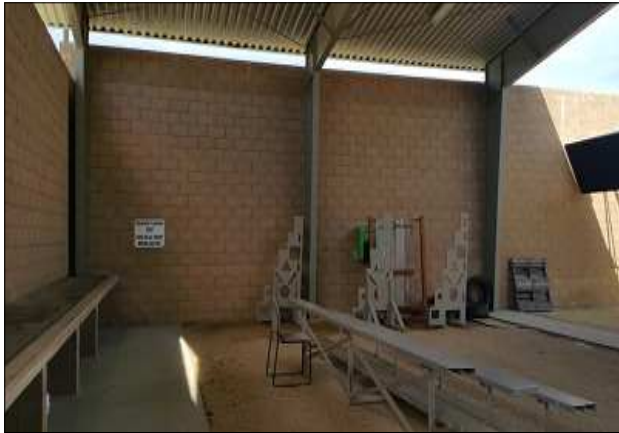
Fig. 3. shooting range facility
