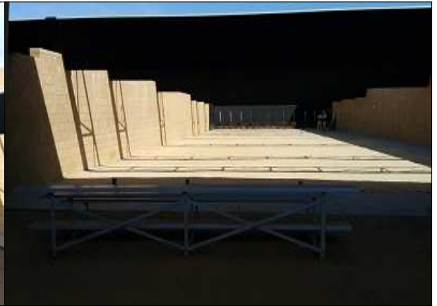
Fig. 4. shooting range facility
