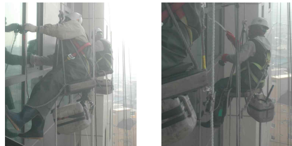
Figure 2. Examples of window cleaning using rope(5)
