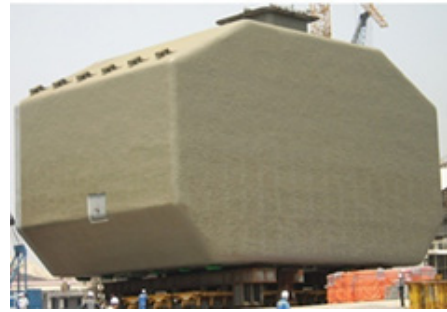
Figure 2. LPG tank insulation (polyurethane spray, combustible).
