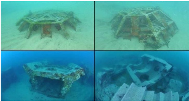
Fig. 1. Buried and broken artificial reefs located in Gangwon. (Data: https://blog.naver.com/withwanju/220834133129 )
