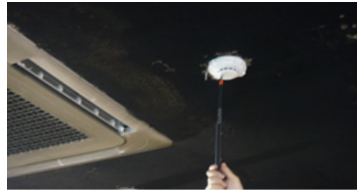
Figure 5. Measuring wind velocity of air conditioner.
