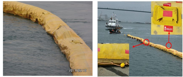
(a) Before improvement (b) After improvement
