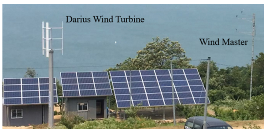
Fig. 1. Picture of test station 9)
