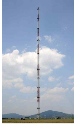
Figure 2. Boseong Meteorological Observation Tower
