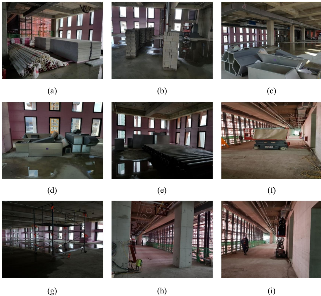
Figure 10. Communication-interfering elements for indoor construction sites: (a) mortar, PVC pipes, and gypsum board; (b) bricks; (c) ducts; (d) ducts; (e) metal pipes; (f) rental equipment; (g) scaffolding; (h) structural columns; and (i) structural walls.
