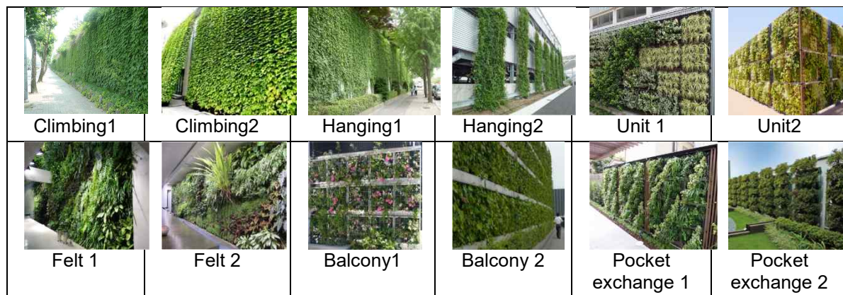
Figure 2. Pictures of 6 Construction Method of Green Wall
