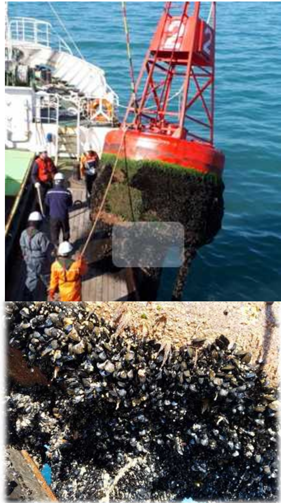
Fig. 2 LL-26(M) type buoy lifting work(top) and attached shellfish(bottom)
