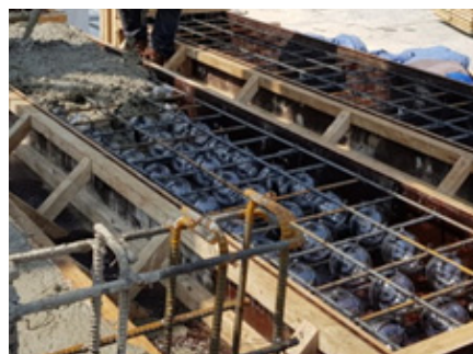
Fig. 1. Production of Hollow Core Specimens
