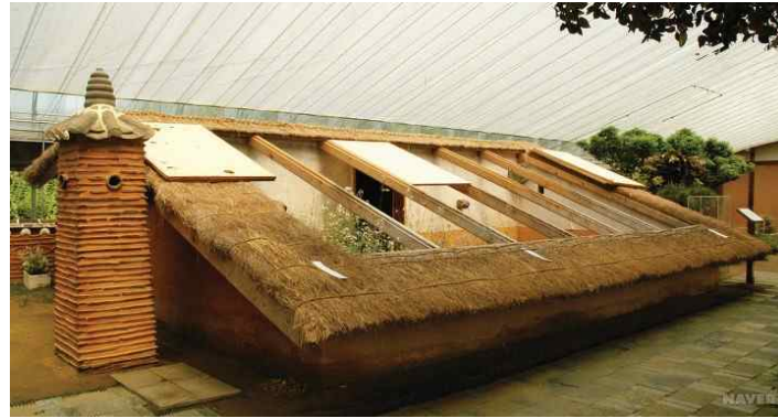
Figure 2. Reproduction of a greenhouse in accordance with the “Dongjeolchae” greenhouse construction
