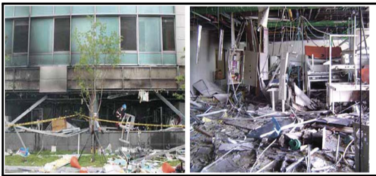
Fig. 1. Damage caused by gas explosion pressure[1].
