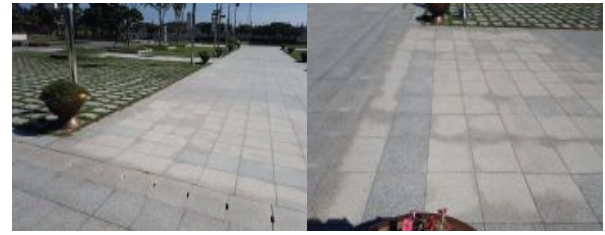
Fig. 5 Test site for installation of concrete block
