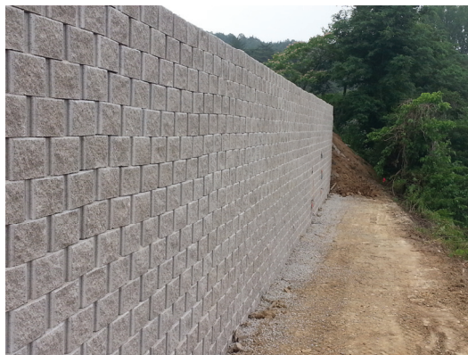
Photo 1 Reinforced soil retaining wall
