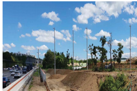
Fig. 2. Picture of Noise Meter Installation
