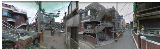
Fig. 3. old residential area
