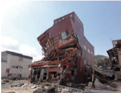
Photo 2. Damaged building due to the ship collision
