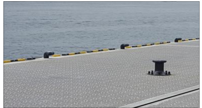
Fig. 2. Photo of bollard and bitt (Port of Busan).
