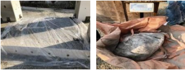
Fig. 11. Measurement of rebounded shotcrete
