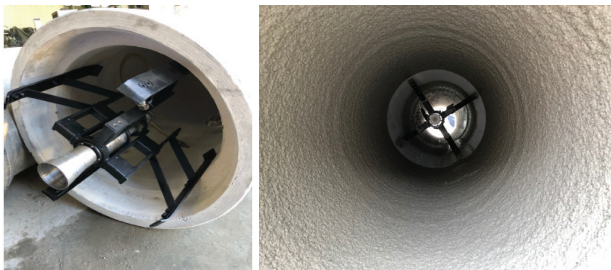
Fig. 1. Construction image of glycolix coating materials by the lining technique
