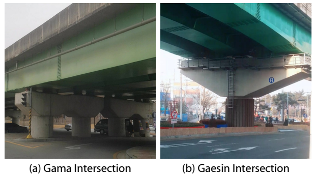
Fig. 4. Steel Box Girder Bridge
