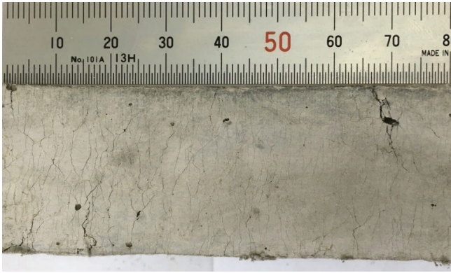
Fig. 10 Crack patterns formed on a specimen with Mix 6
