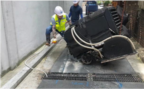
Fig. 16. Rotation of eco-friendly road cutter
