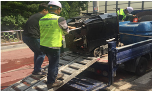
Fig. 17. Loading eco-friendly road cutter
