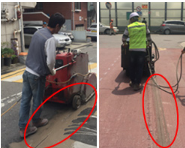
Fig. 18. Comparison of the amount of cutting slugs generated by the two cutters
