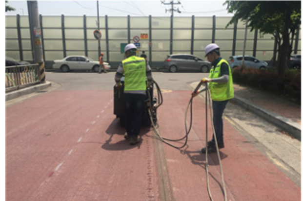
Fig. 14. Road cutting with eco-friendly road cutter
