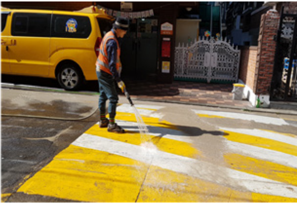
Fig. 11. Water cleaning on site
