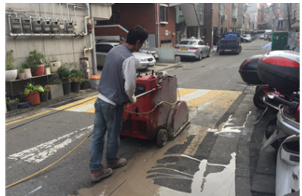
Fig. 9. Road cutting with low noise road cutter
