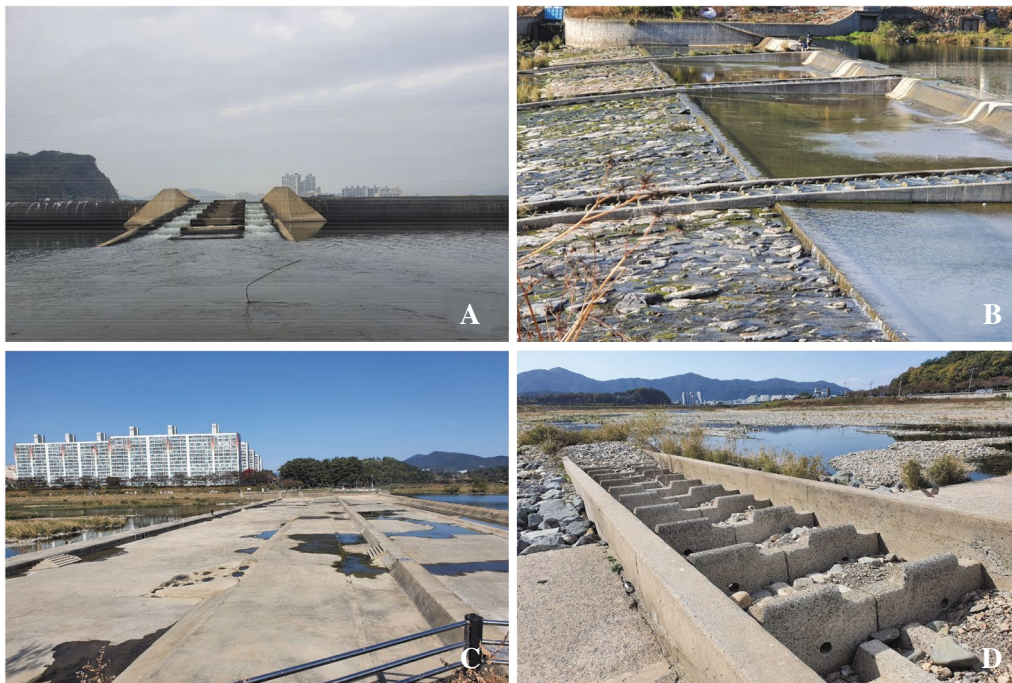
Appendix 2. Weirs in Milyang River (Physically possible for upstream migration (A, B), Physically unable to go upstream (C), Physically possible, but impossible due to lack of flux (D)).
