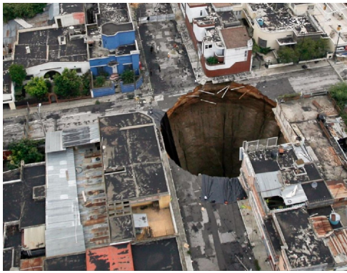
[Fig. 1] Massive sinkhole disaster in urban area, Guatemala, 2007 [2]
